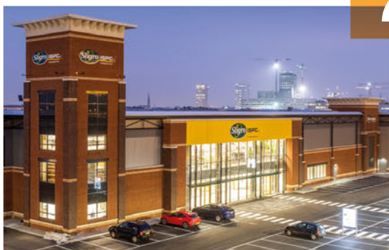
Opened in 2018 in Antwerp, the first Sligro cash-and-carry outlet and wholesale delivery service in Belgium.
